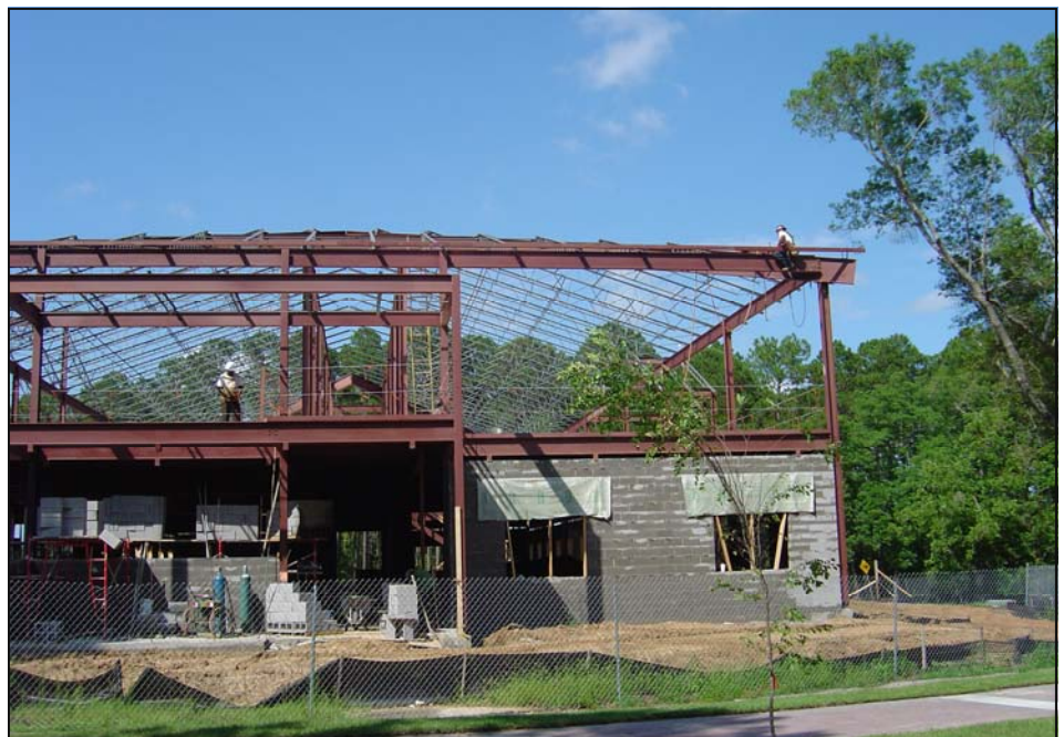
Construction is ahead of schedule on the new Health Sciences Building.
